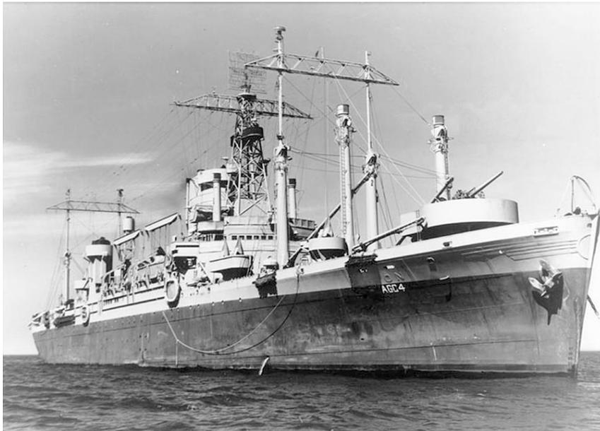
*SS Ancon as USS Ancon (AGC-4) at anchor in Chesapeake Bay in May 1943, after conversion from a troop transport to an amphibious command ship (AGC). Note that some of her civilian bow ornamentation, although painted over, is still visible. US Navy photo # NH 95389.*
